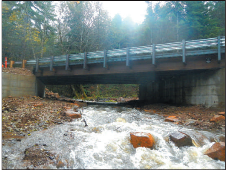
Bridge installed on Clatskanie River at Schaffer Road.
