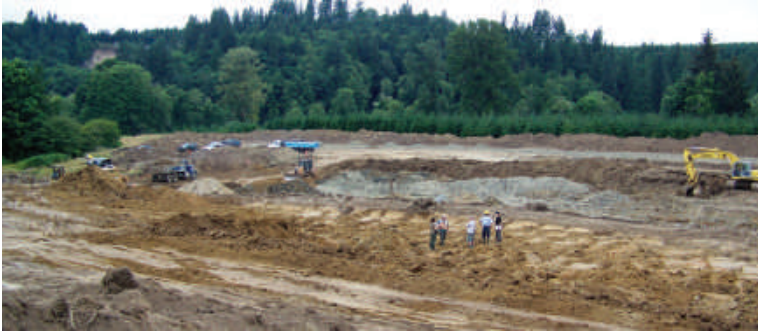
LEFT: Construction crews build the Fleming pond, August 2012.
