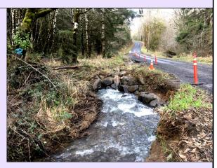
and floods the public road at high flows. This project will remove the culvert and replace it with a larger structure to open up about 2.8 miles of Essential Fish Habitat (EFH) for ESA listed Coho Salmon as well as Steelhead for high quality spawning and rearing grounds.
