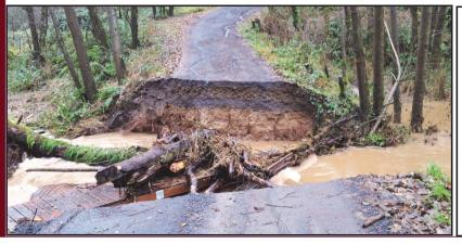
Extreme damage to Hills Haven Road in Deer Island during the December 2015 storm cut off several residents from their homes. Repairing the road, installing a new culvert, and stabilizing the streambank along Merrill Creek is one of the 14 emergency projects the District is overseeing this year.
