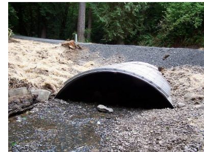
Cox Creek Culvert After
