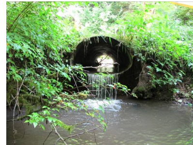
Cox Creek Culvert Before
