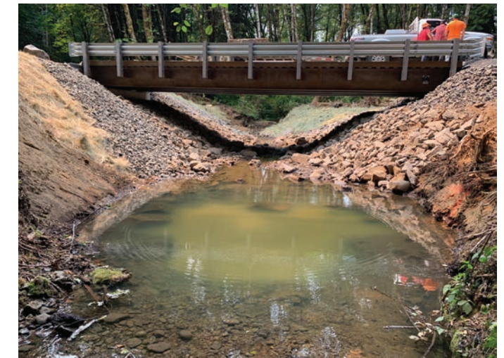
Photo bottom After: Brush Creek bridge
