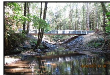
Pebble Creek - Completed Bridge
